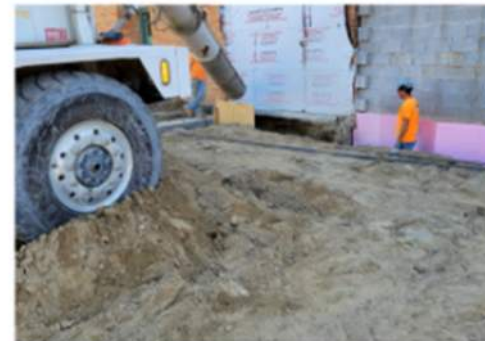
Exterior Foundation Install
