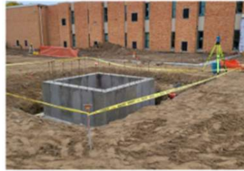
Elevator Pit Foundations
