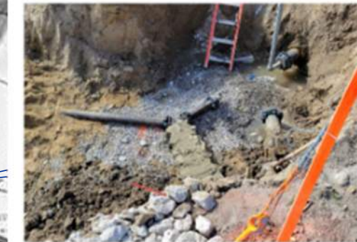
Water Main Install
